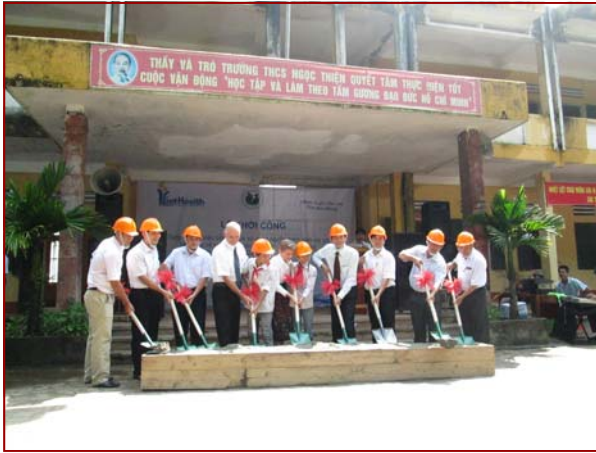
Donors and district officials break ground on the project, which will bring toilets to eleven district schools.
