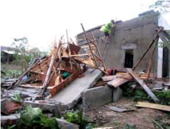
A local house damaged in Quang Binh province (Source: Thanh-Nien News)
