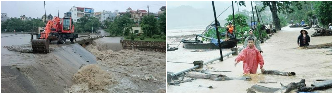
Left: The accumulated rainfall during the 1- 2 Aug in Uong Bi town, Quang Ninh, has caused very high flooding. A spillway (dam) was broken down to release the flood pressure in Uong Bi (Vietnamnet)
