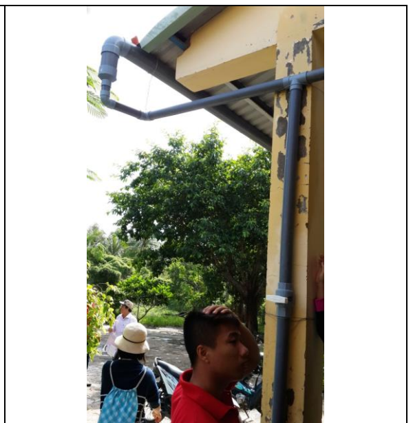
New version of gutter and connecting pipes in Ca Mau
